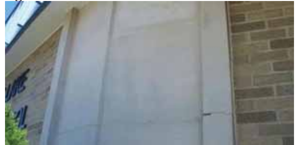
Figure 12 - Precast Joint Crack
