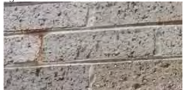
Figure 15 - Joint Reinforcement Corrosion
