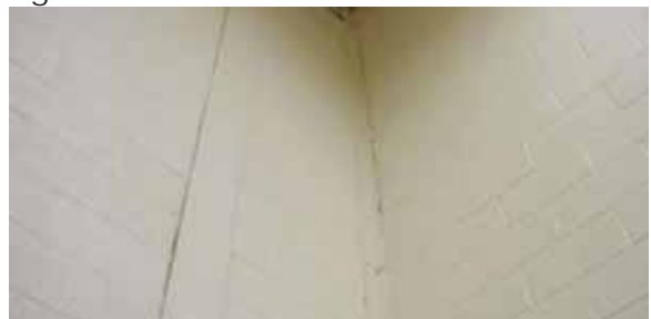
Figure 10 - Crack at CMU Joint
