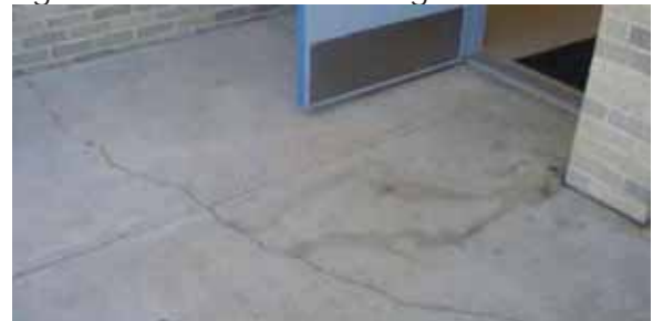
Figure 18 - Sidewalk Cracking
