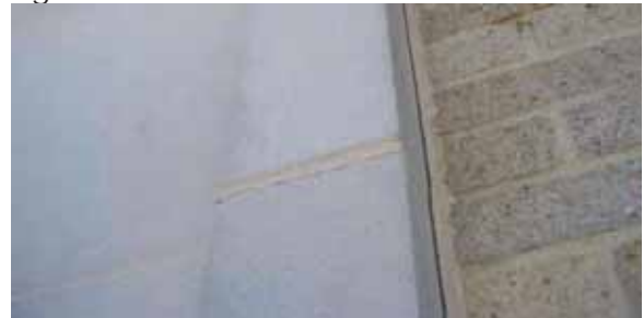
Figure 13 - Mortar Crack at Precast
