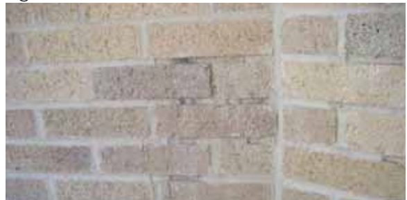
Figure 4 - Mortar Erosion
