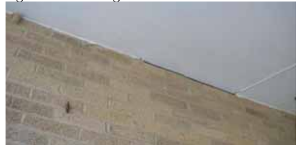
Figure 17 - Missing Caulk at Soffit
