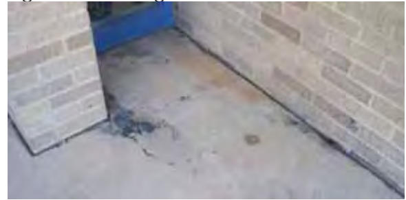
Figure 16 - Missing Caulk
