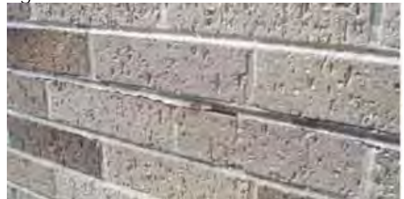
Figure 14 - Joint Reinforcement Corrosion
