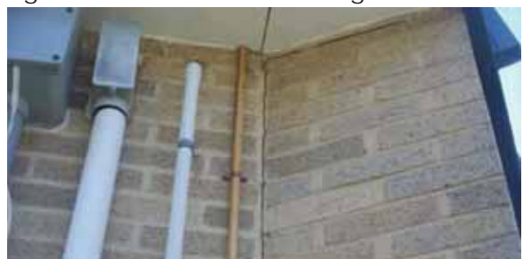
Figure 5 - Mortar Joint Cracking
