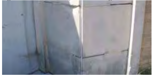
Figure 6 - Precast Impact Damage
