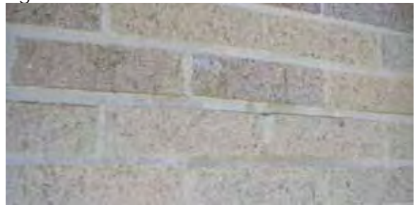
Figure 8 - Mortar Joint Crack
