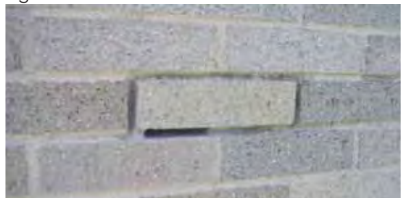
Figure 5 - Mortar Joint Cracking
