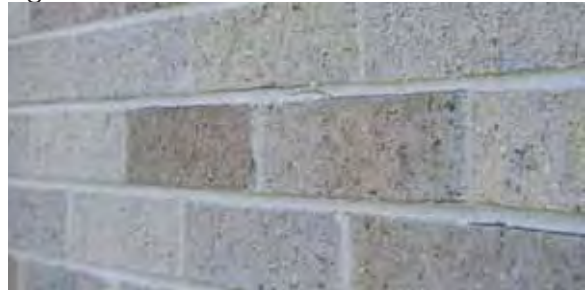
Figure 7 - Mortar Joint Crack
