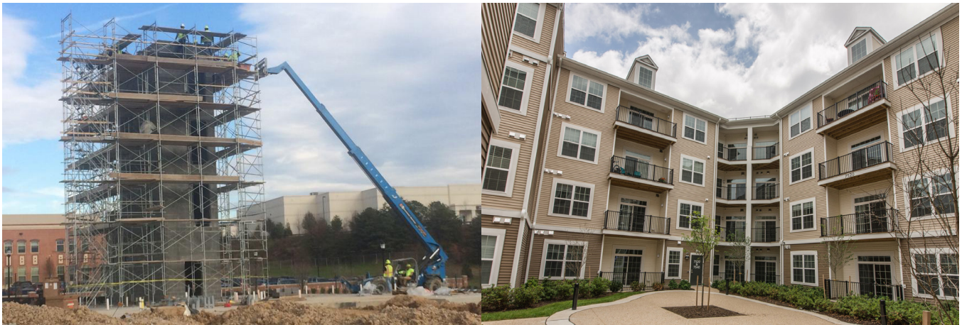
Oxford Square construction.
