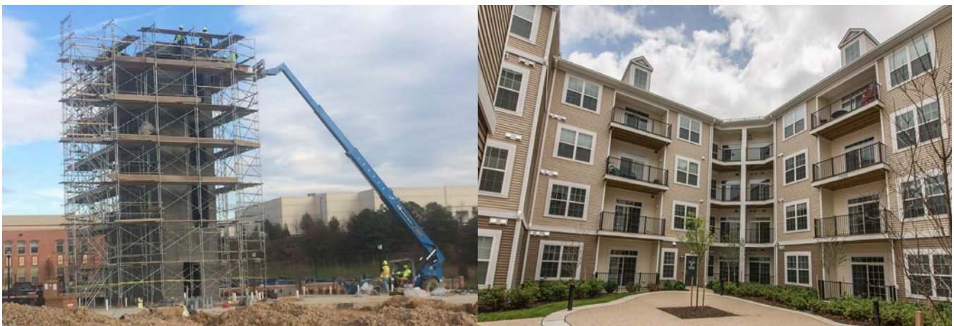
Oxford Square construction.
