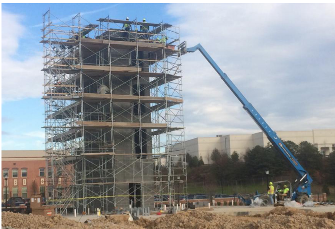
Oxford Square construction.
