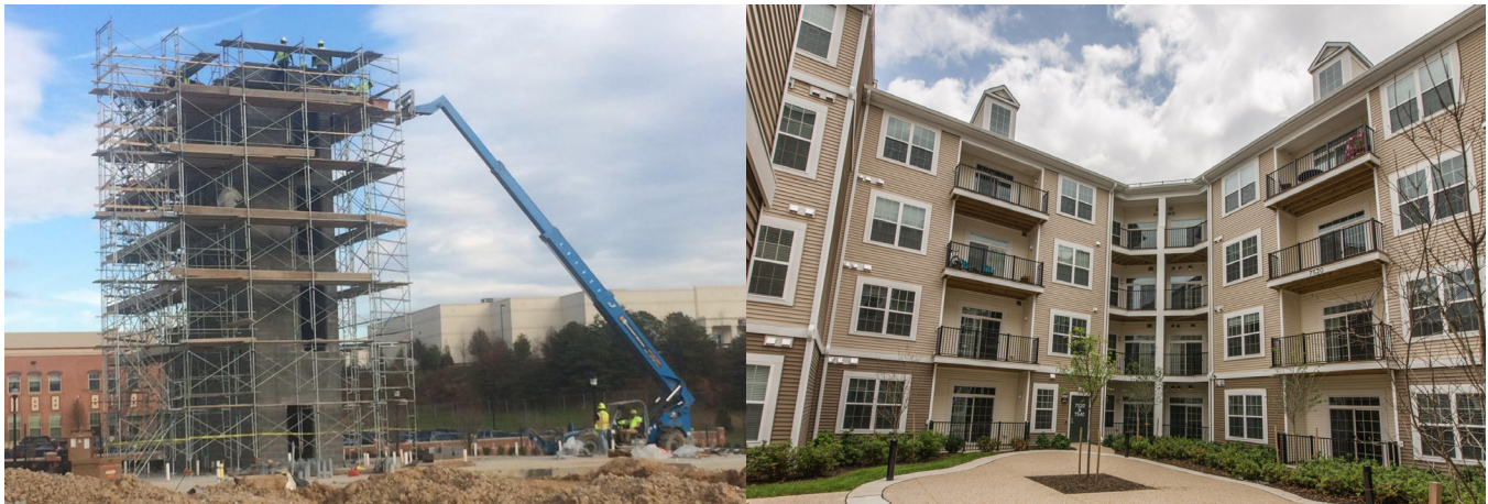
Oxford Square construction.
