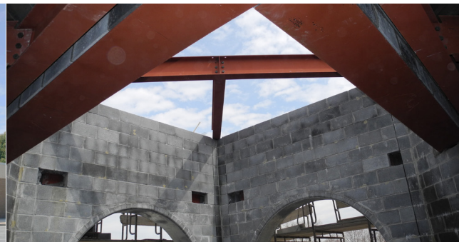
Atholton HS presently under renovation.
