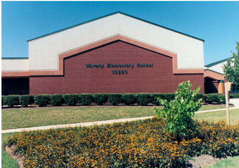
The second phase addition to Waverly ES will help relieve crowding in the Northern Region.
