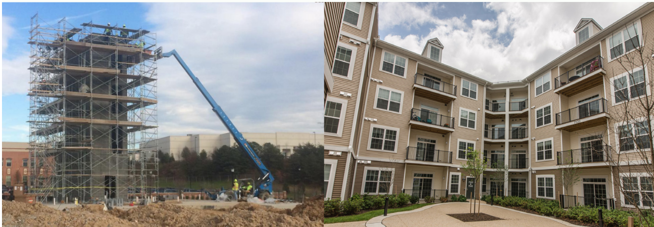
Oxford Square construction.
