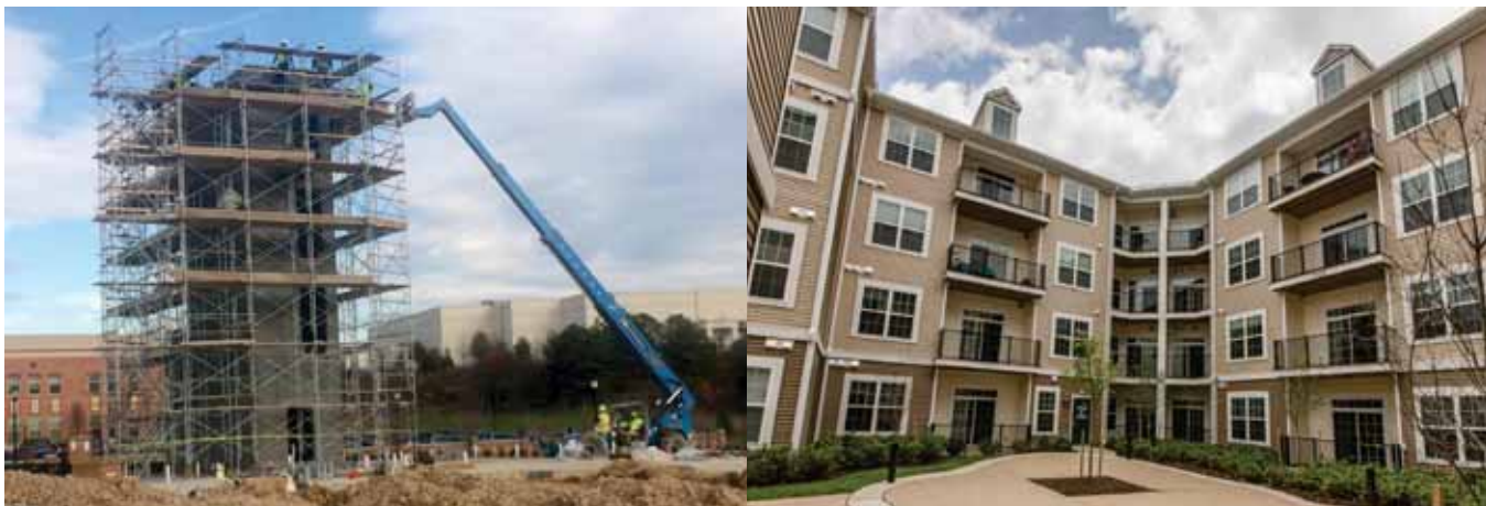
Oxford Square construction.
