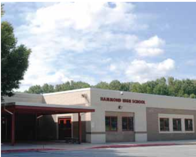
Hammond HS serves the Southeast Region.
