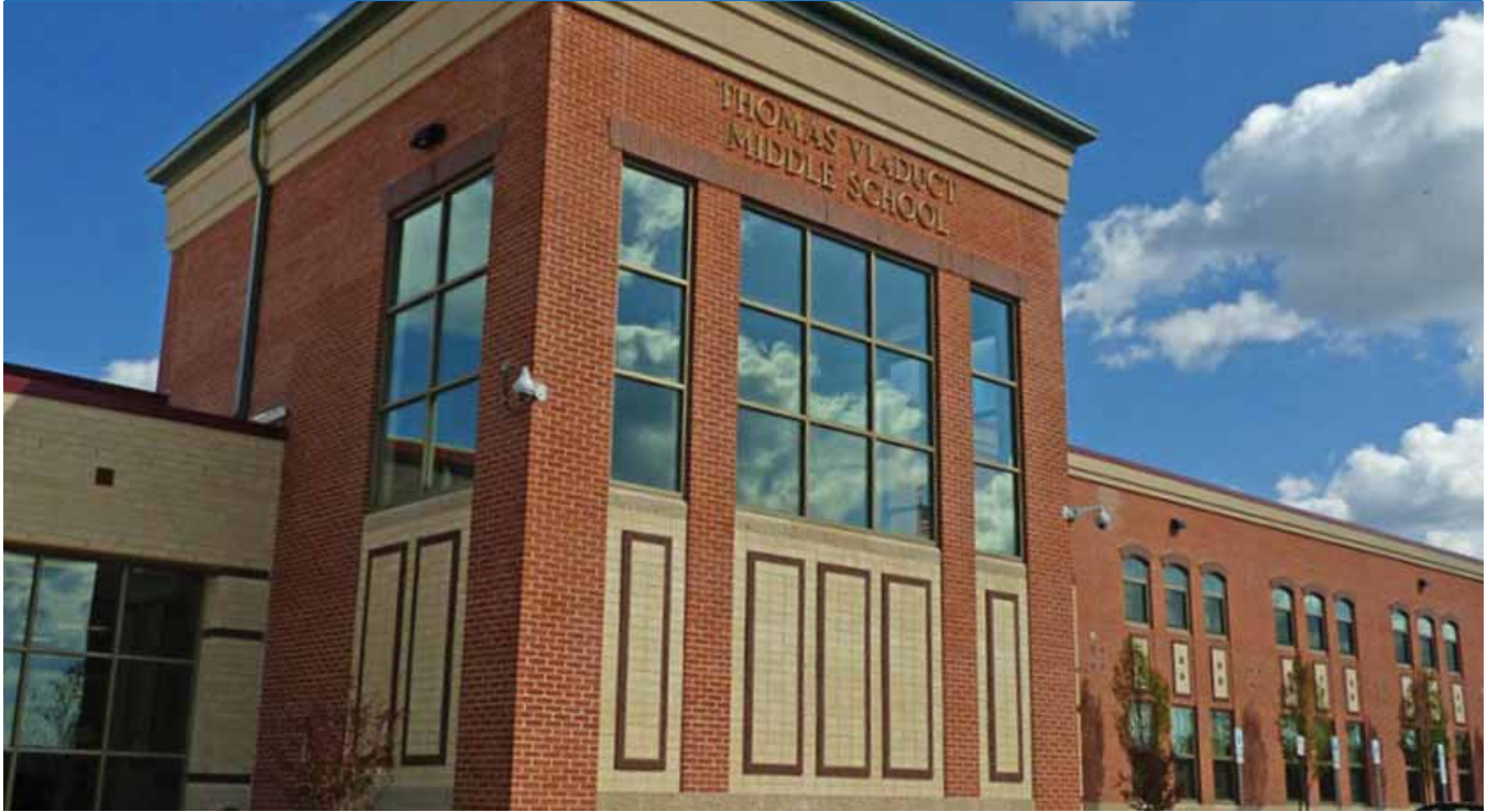
Thomas Viaduct ES opened in August of 2014
